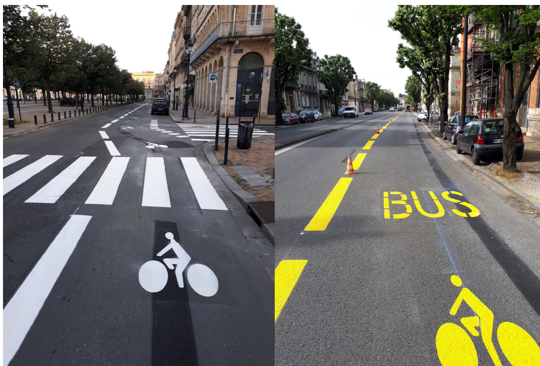
Figure 5. Right: boulevards de Bordeaux, creation of bus/cycling lane, Left: allées de Tourny, Bordeaux, enlargement of existing cycling lanes.
